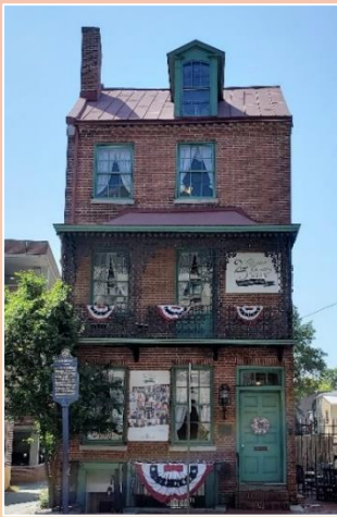
The Lincoln Building 28 West Market Street West Chester, PA 19382 www.chescocf.org www.culturechesco.org
